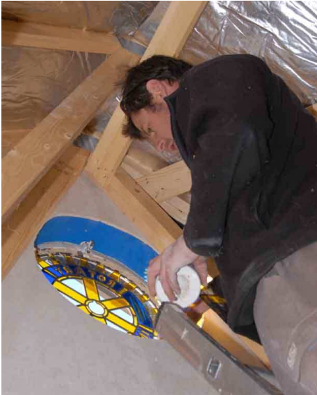
Our carpenter, Vince Smith, fits the Rotary Window that he made for the new building
